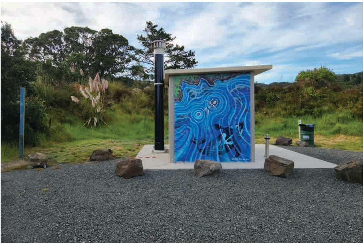
Figure 4. View east of new toilet block. Photo scale = 0.5 m.
